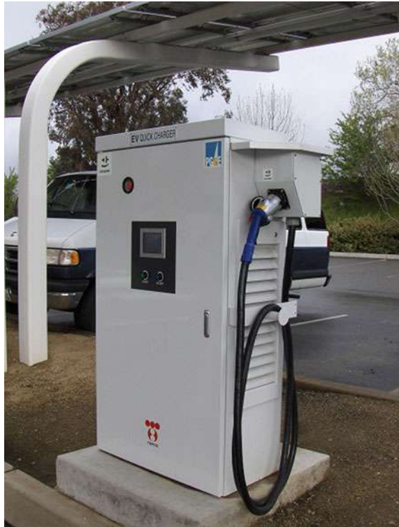
Fig. 3.8 CHAdeMO high-speed charger at Vacaville, California Park and Ride lot (Picture from C-CarTom (Own work) [CC BY-SA 3.0). http://creativecommons.org/licenses/by-sa/3.0 ) or GFDL)
