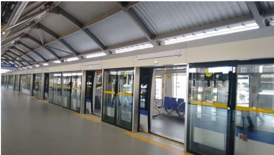
Fig. 1.2 Implementation of platform doors controlled by the signaling system removes operational uncertainty and allows for unmanned metro operation. Source Author
