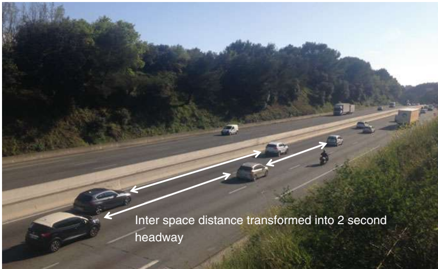
Fig. 4.4 Traffic flow on highway will be influenced by lane width and lateral clearance, the mix of heavy and light vehicles, as well as the human factor. Source Author
