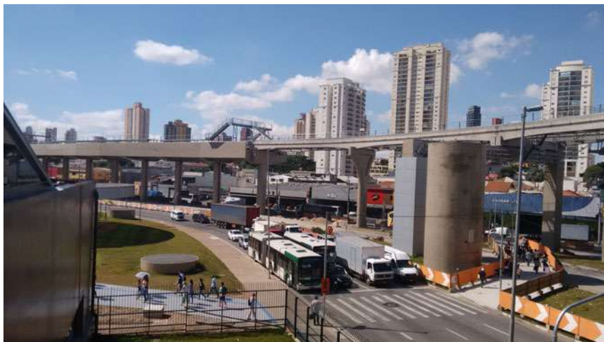
Fig. 4.13 Picture of monorail tracks in the city of Sao Paulo laid between the two lanes of a large avenue, resulting on minimum expropriation and land appropriation. Source Author
