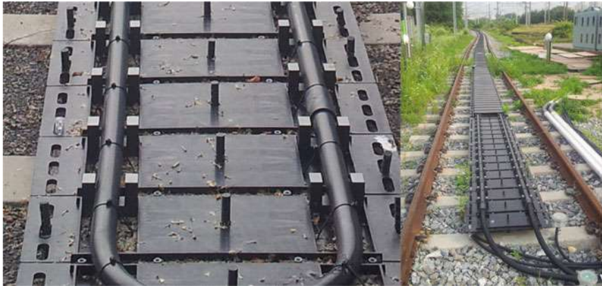
Fig. 17.8 Photographs of developed 128-m transmitter track
