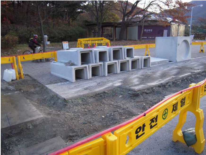
Fig. 11.4 Cutting work of selected road
