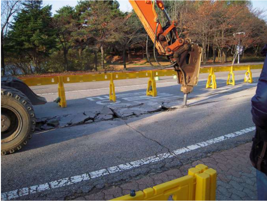
Fig. 11.5 Process for excavating existing road
