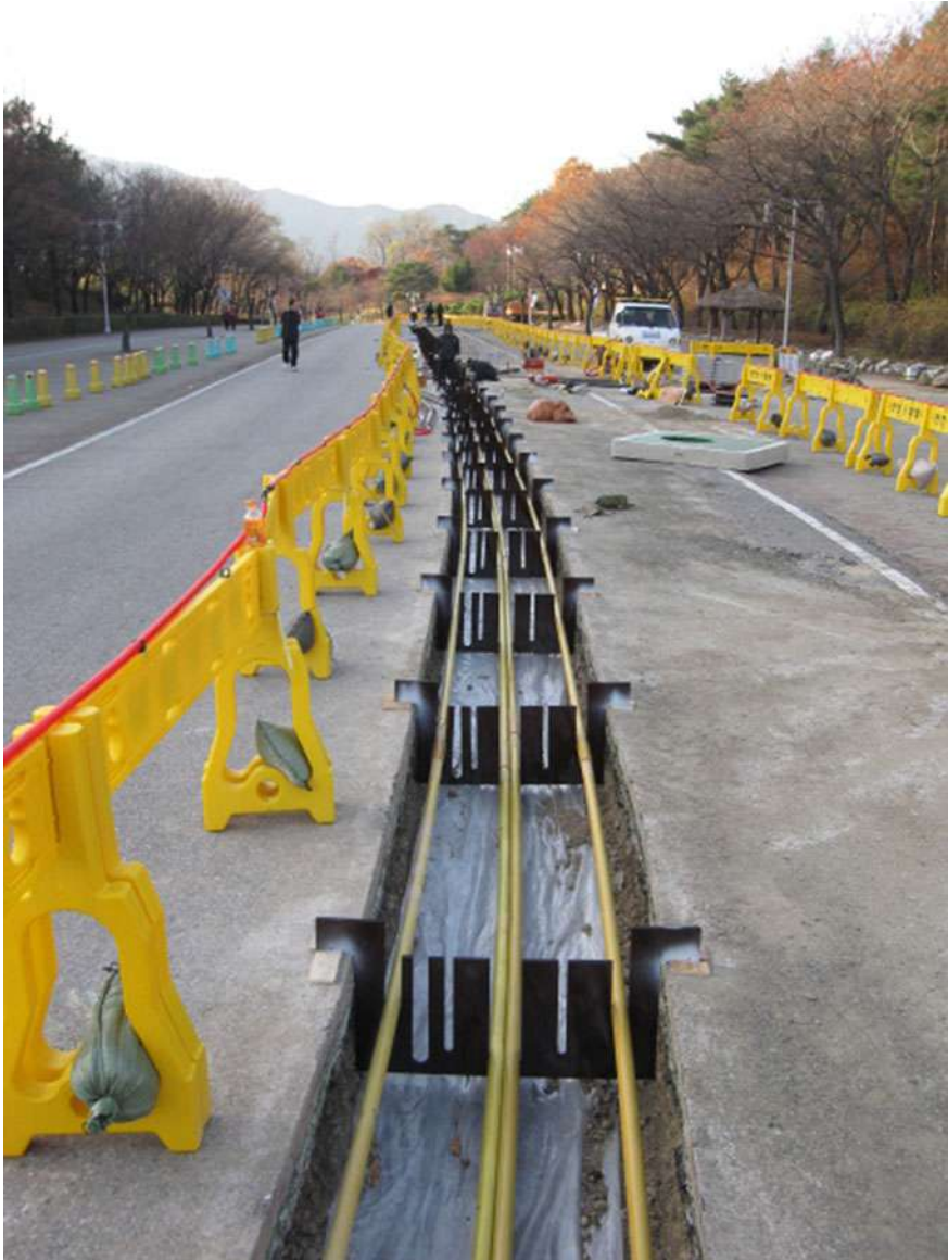
Fig. 11.6 Structure prepared to install power supply system
